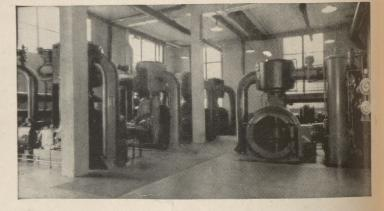
. installation of five "XVHE-2" Synchronous Motor-Driven units compressing air for the operation of forging hammers and many other purposes in the manufacture of high-speed alloy and stainless steels.
