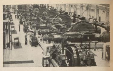
. . five 2500 hp 5000 PSI gas compressors installed in a Canadian synthetic ammonia plant.
