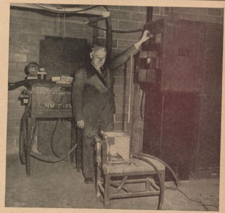
**PROF.** J. U. MacEWEN, chairman of the department of Metallurgy, is shown here regulating the power of an Ajax 20,000-volt conduction furnace for rapid melting of metals and alloys. It can melt 30 pounds of steel in one hour. It has a practical top temperature of 1,700 C.
