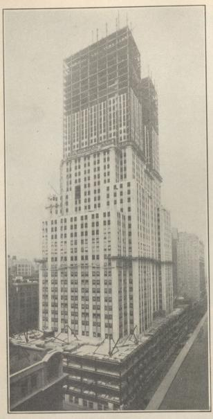
JULY 31, 1930 Four months from the date of the first photograph of our series, steel was up to the 47th storey, masonry to the 30th storey, and the chrome steel window trim to approximately the 38th storey.
