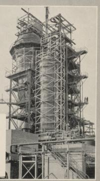
Left: Imposing towers of Polymer Corporation's synthetic rubber plant at Sarnia, built by Dominion Bridge. One of these is 165' 4" high and is the largest ever built in Canada.
