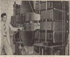
Here is the magnet of the 70,000,000 electronvolt-synchroton installed at Queen's University for the purpose of X-ray and nuclear research. It was built and erected under the supervision of General Electric's nucleonics engineers.
