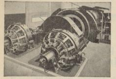
Mine hoist driven by two motors totalling 4500 hp. Electric motors increase the output and earning capacity of workers.
