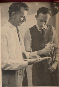
Aluminum "paint" is sprayed on foamed plastic to produce a light substitute for glass in electromagnetic lenses. With student Harald Moen, Viscount, Sask., holding a plastic sheet, is Dr. Bekefi.
