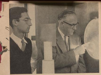
Prof. Woonton, Laboratory Director, explains to student Issie Shkarofsky, Montreal, the passage of microwaves through a solid plastic lens and the measurement of those reflected back to the source by a metal plate.
