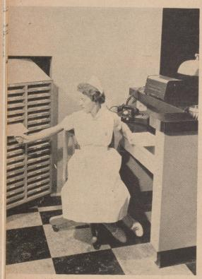
A head nurse's station is a model of efficiency. When the patient touches a switch, a light shows in the box on top of the desk, identifying the bed in the nursing unit. The nurse answers on the telephone. A sensitive microphone in the wall adjoining the bed enables conversation between patient and nurse, cutting walking time by 50 per cent for the nurse.
