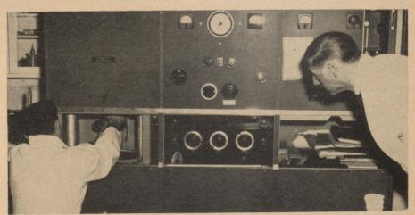
This is a view of the optical analytical ultra-centrifuge. Dr. Alec Sehon is adjusting the rotor which spins at 60,000 RPM while Dr. Bram Rose looks on. As the spinning progresses, the migration of the small protein particles in the gravitational field cause them to separate, the heavier ones moving faster than the lighter ones. The actual process is photographed in this machine by a complicated system of lenses.
