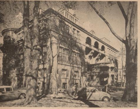
"The Physics Building . . . in order to avoid magnetic interference, no iron or steel was used ... probably one of the last big buildings constructed entirely of wood and masonry in Canada."
