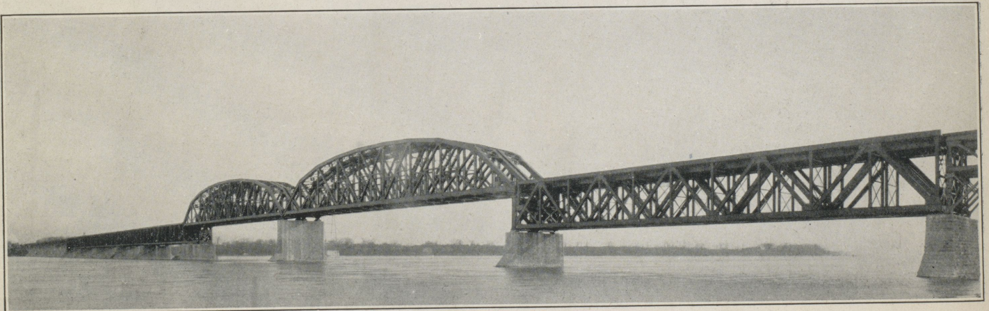
Photograph, courtesy Canadian Pacific Railway The Canadian Pacific Bridge across the St. Lawrence River at Lachine, Que.
