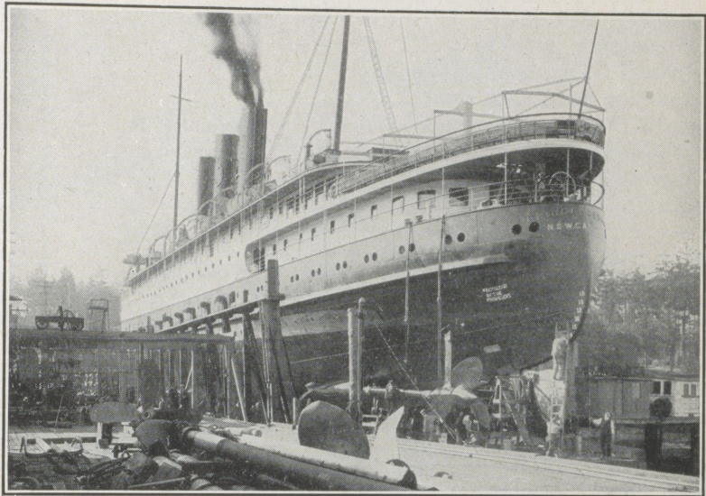
3,000-TON VESSEL ON MARINE RAILWAY
