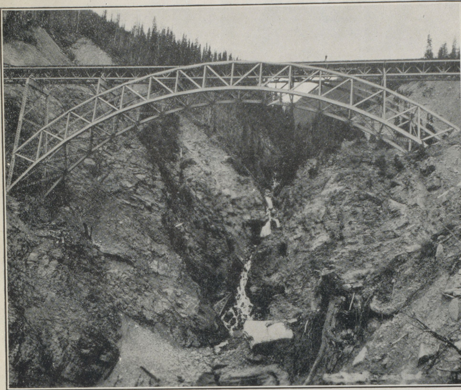
Photograph, courtesy Canadian Pacific Railway This arch bridge over Surprise Creek Glacier is typical of the many structures along the line of the Canadian Pacific Railway in the Rocky Mountains
