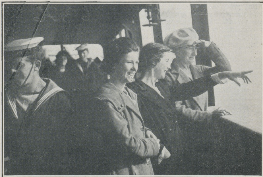
Land in sight at last Photograph, courtesy Canadian Pacific Railway
