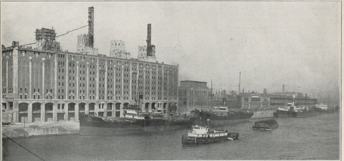
A portion of the Harbor of Montreal, showing recently constructed two-million-dollar cold storage plant. British & Colonial Press Photograph
