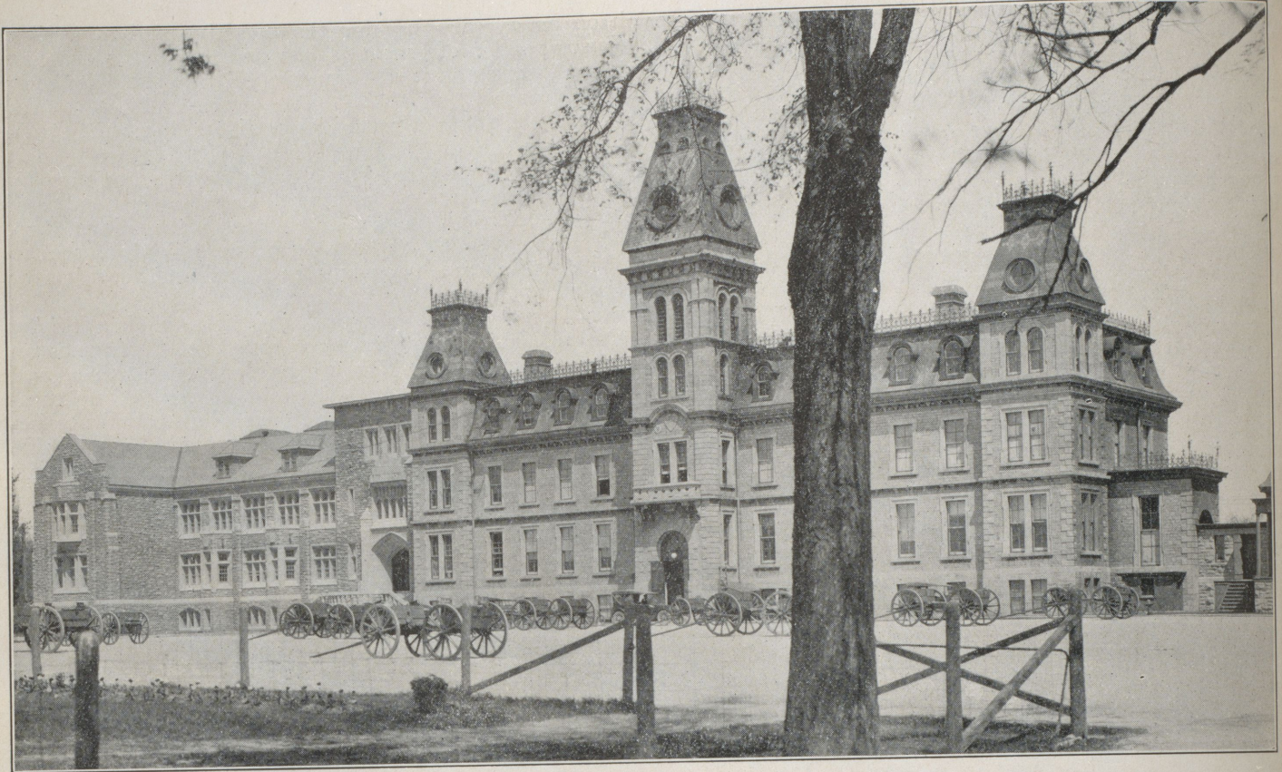
The Main Building of the Royal Military College, Kingston, Ont., showing, on the left, the recently completed Sir Arthur Currie Hall
