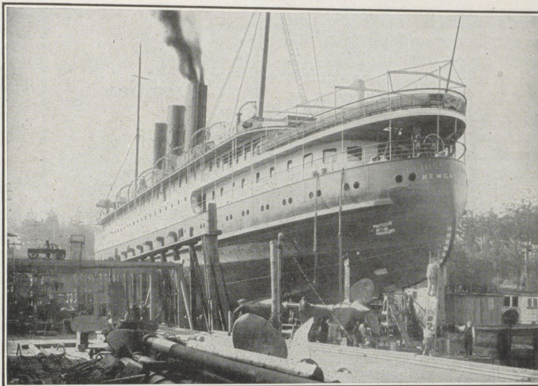
3,000-TON VESSEL ON MARINE RAILWAY
