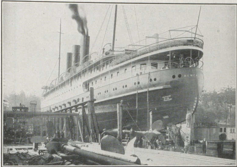
3,000-TON VESSEL ON MARINE RAILWAY
