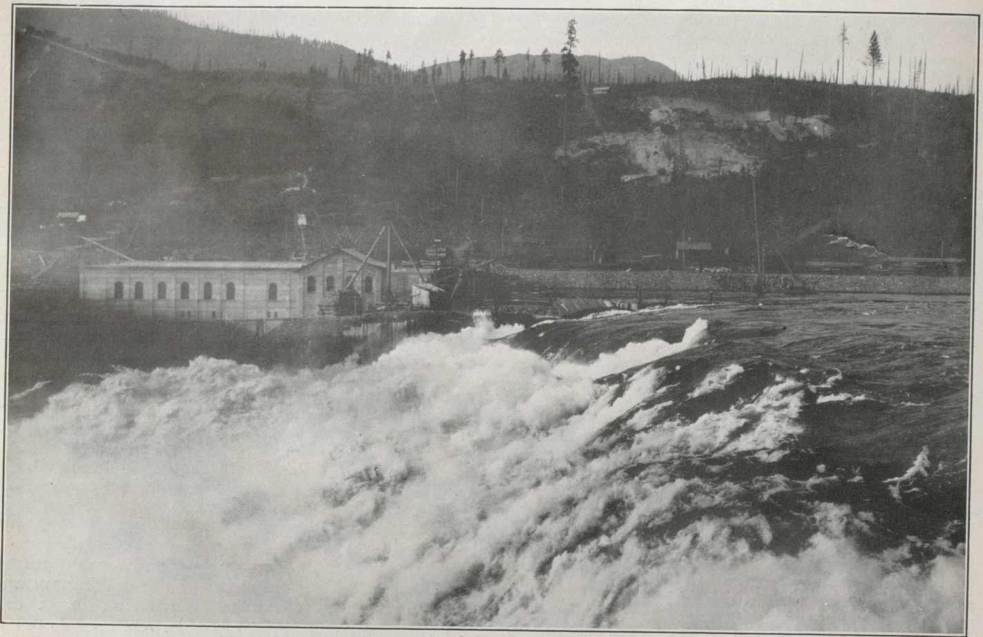
The West Kootenay Power Station, Bennington Falls, near Nelson, British Columbia
