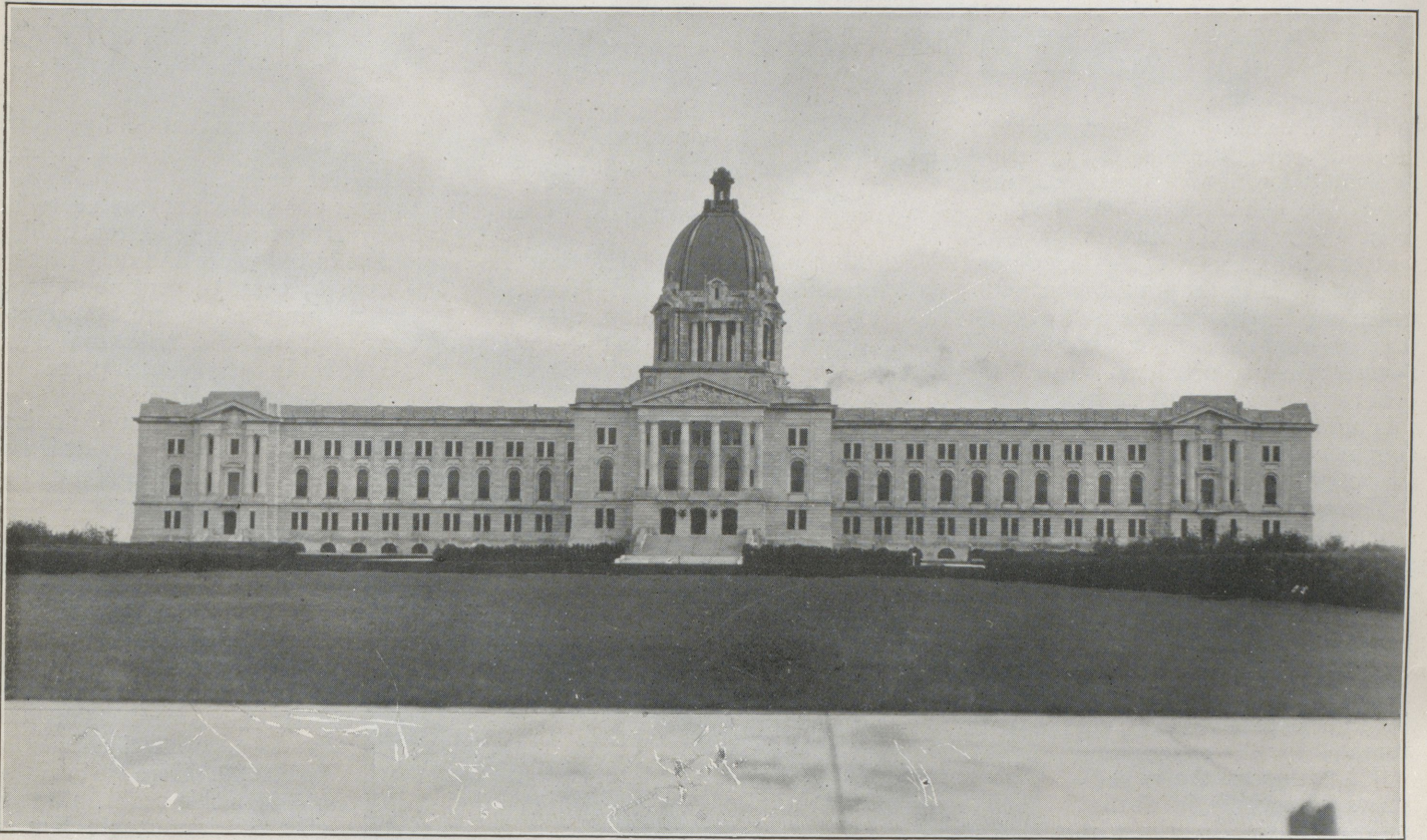
The New Legislative Assembly Buildings at Regina, Saskatchewan, reflect eloquently the growth of the Canadian West British & Colonial Press Photograph
