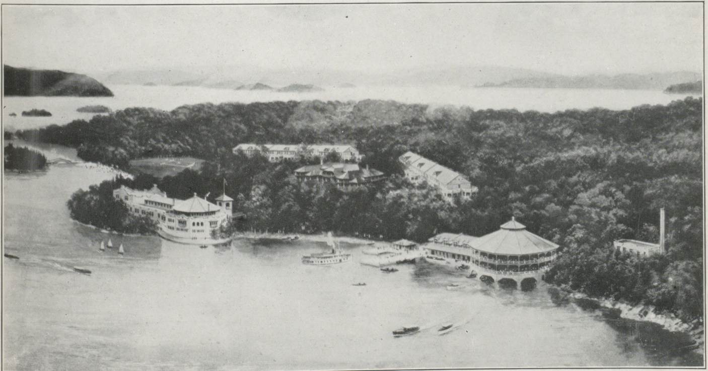
Photograph, courtesy Grand Trunk Railway System
