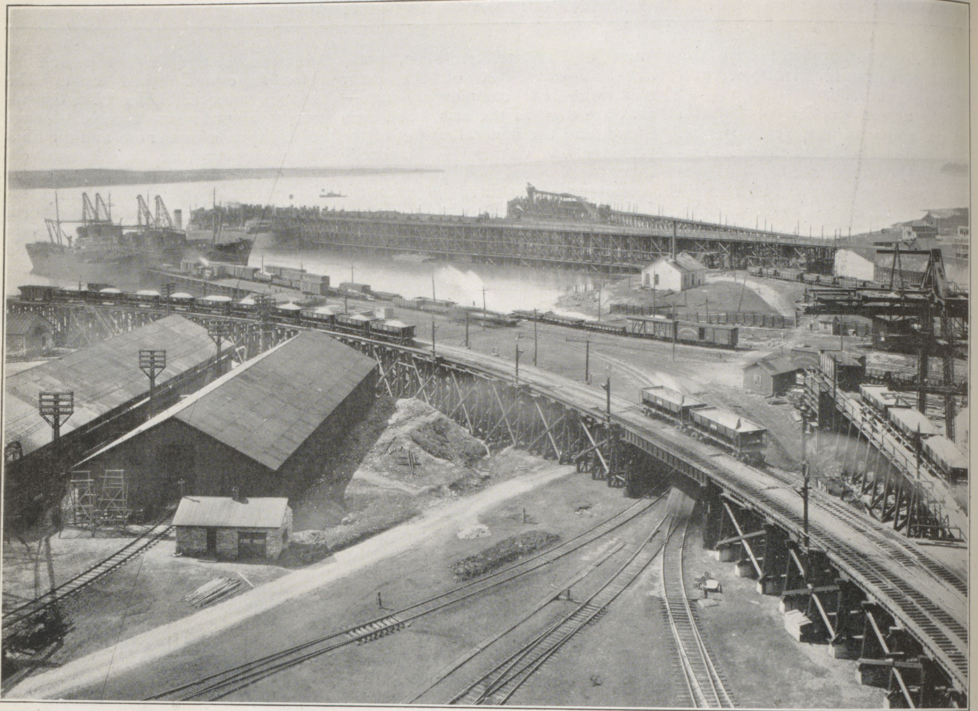
A view of the ore-discharging docks of the Dominion Iron & Steel Company, Limited, Sydney, N. S. Photograph by S. J. Hayward, Montreal
