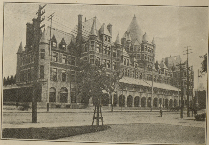
Gare VIGER Station
