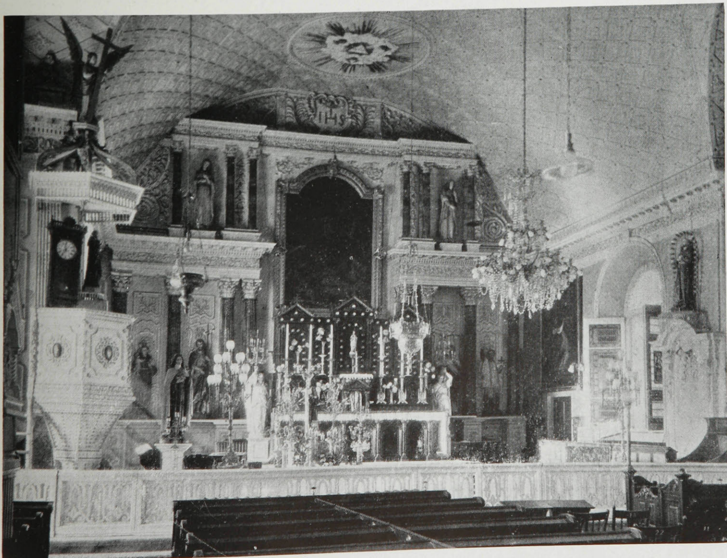
Pointe aux Trembles, Interior. Burnt, 1937
