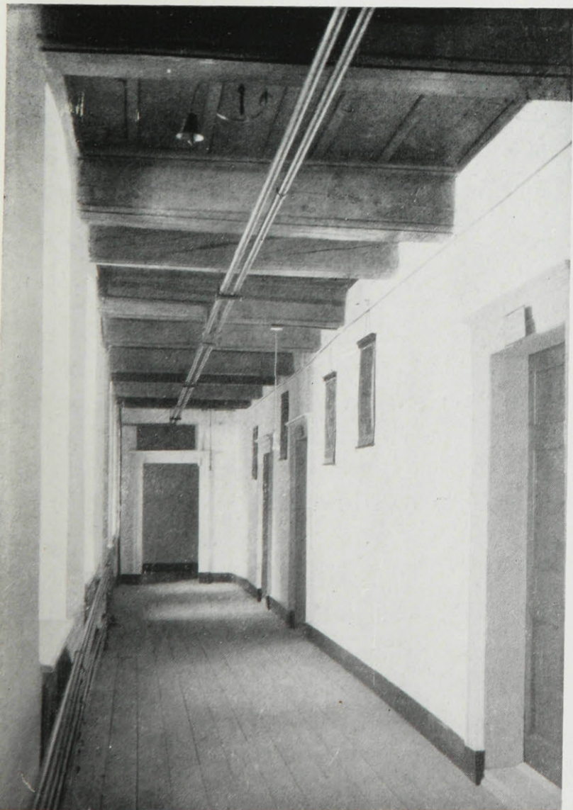
The Corridor on the North Side of the Cloister
