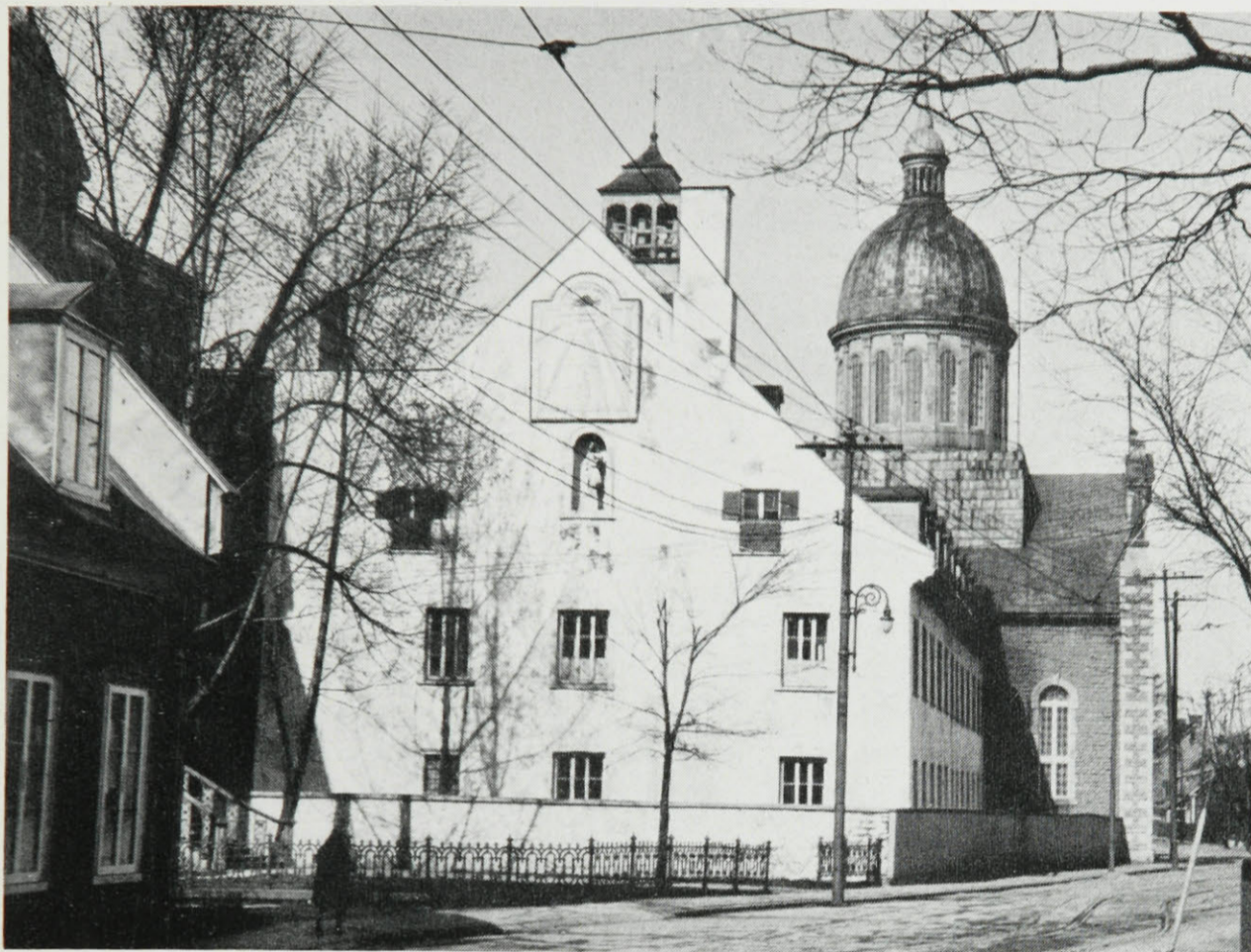
The West Gable
