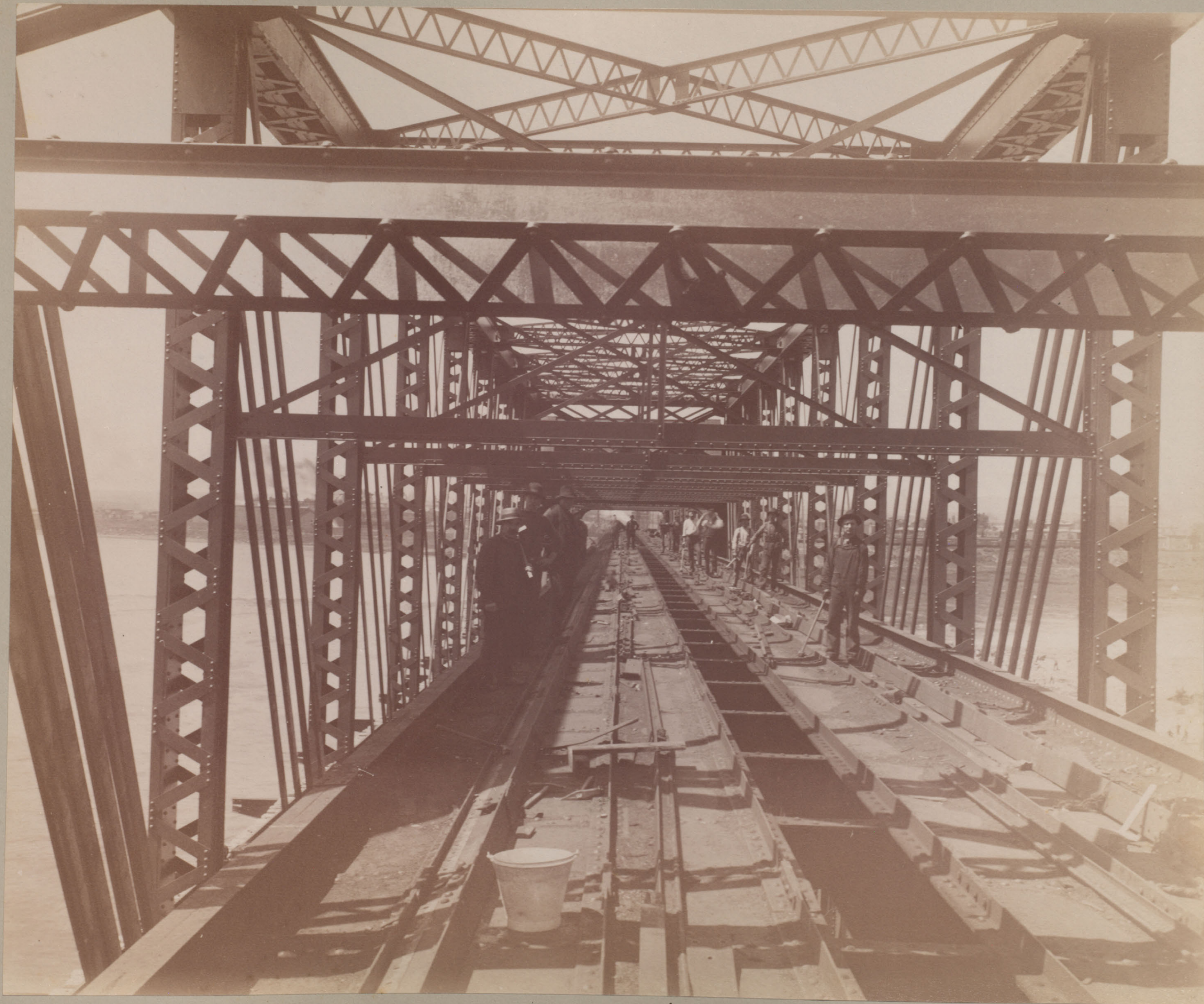
Commencing Removal of Old Tube Top View
