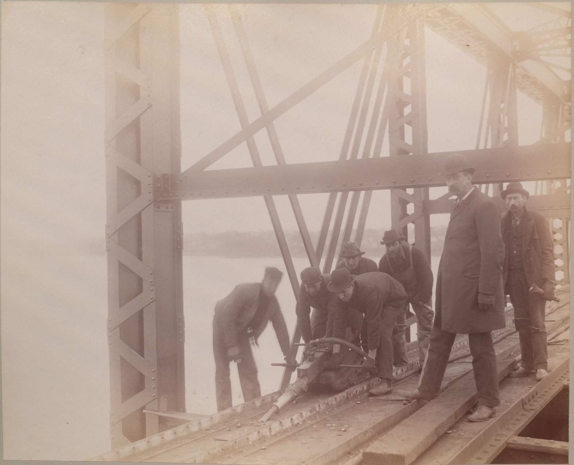
Removal of Tubes - Pneumatic Chisel At Work
