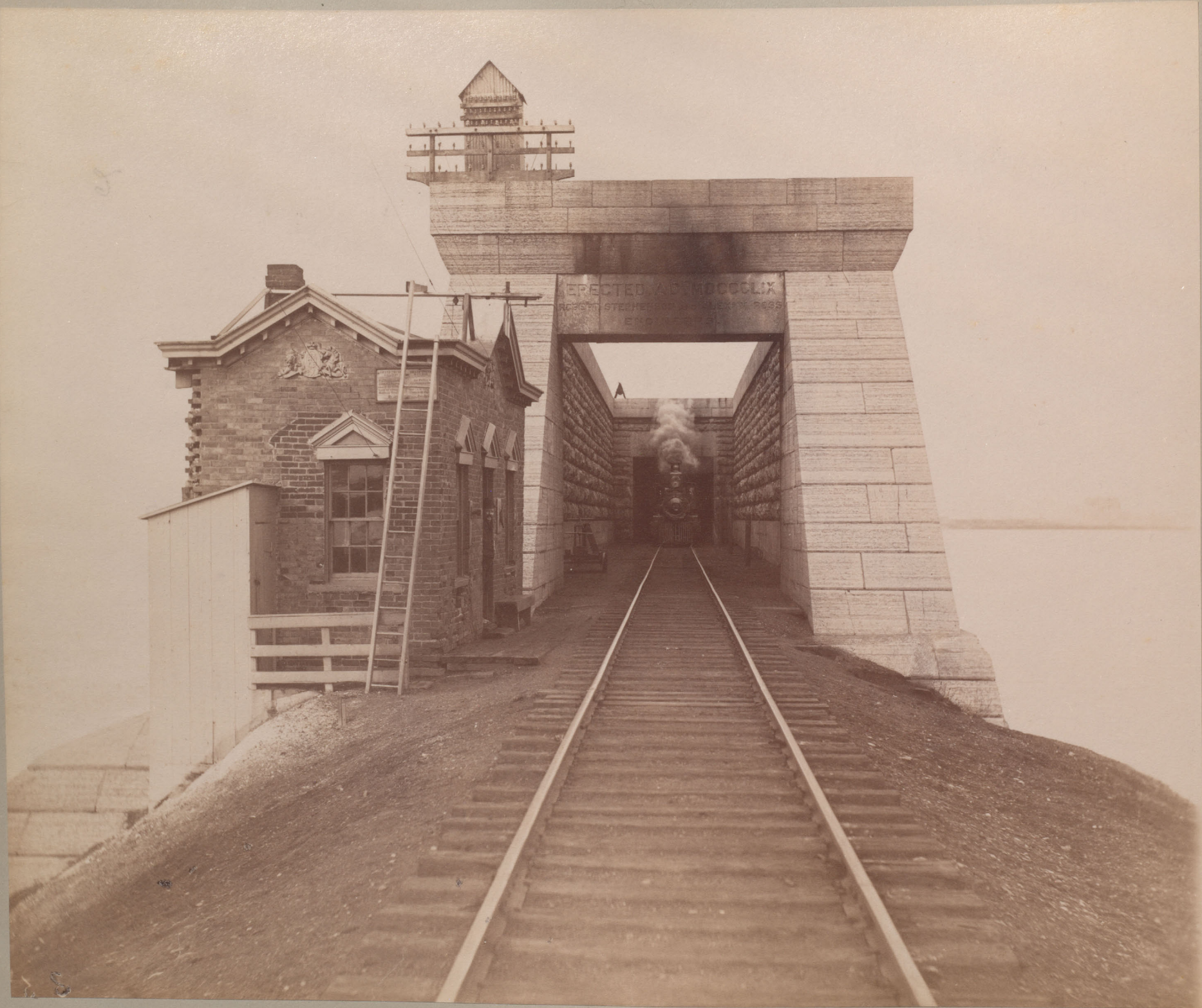
Former Tubular Bridge Easterly Portal 1897
