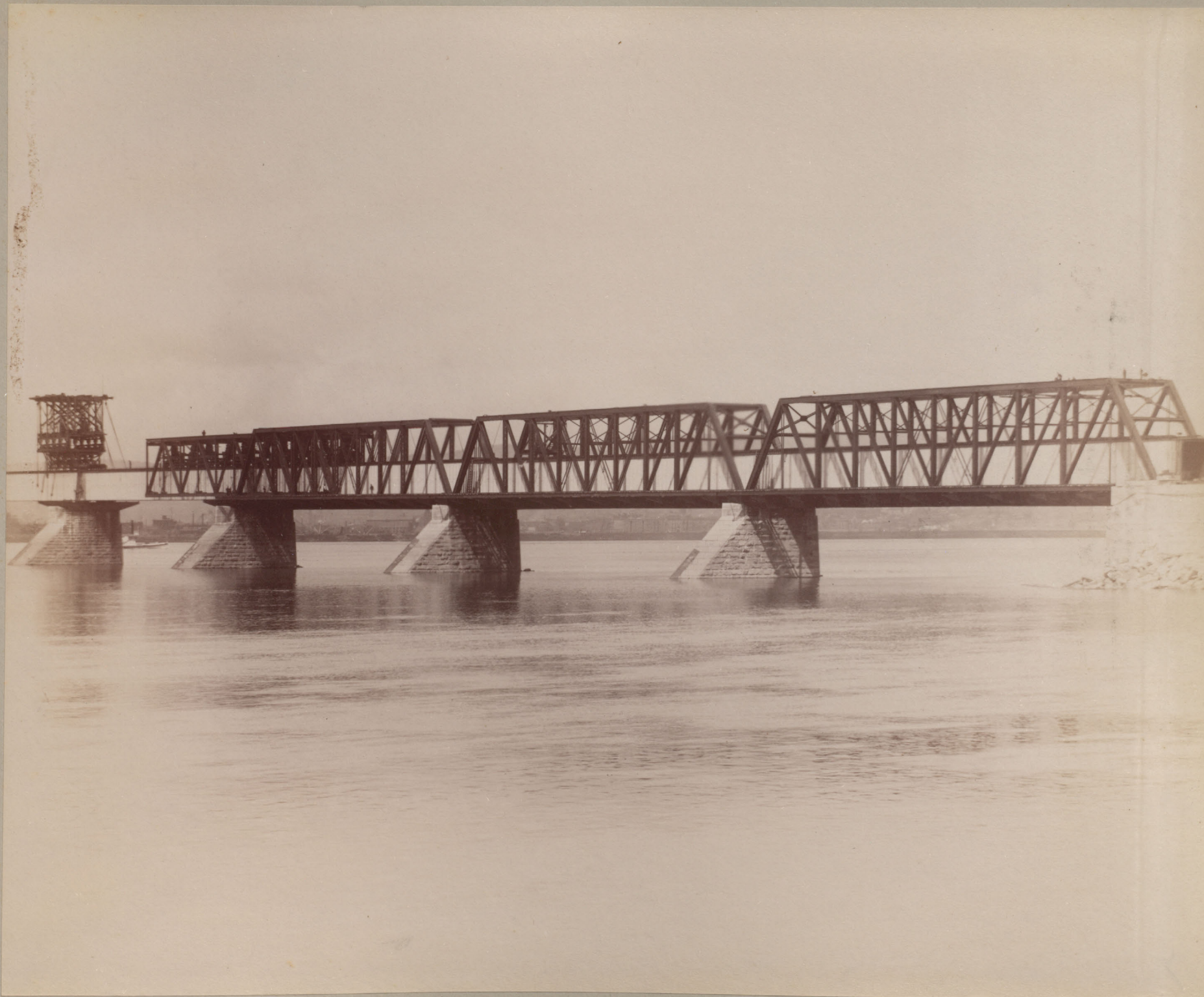
—Erection Truss Moving Over Span 22— —May 28 th 1898—
