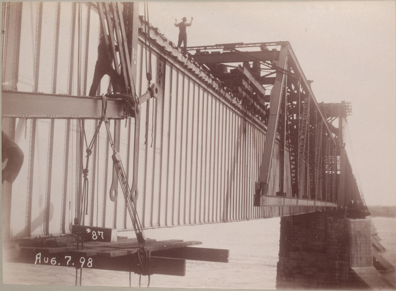
— Moving Erection Truss Over Centre Span — — Aug. 7 th 1898 —
