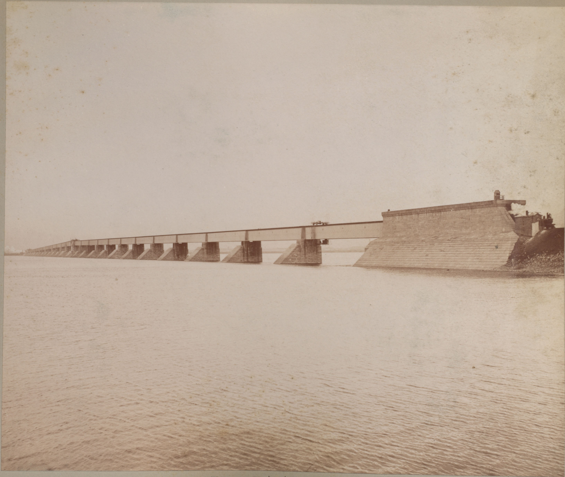
— Former Tubular Bridge — — General View from Easterly Shore — — 1897 —
