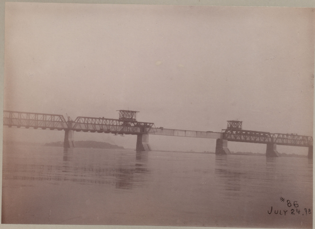
Centre Span previous To Erection Truss Being Moved Over July. 24 th 1898
