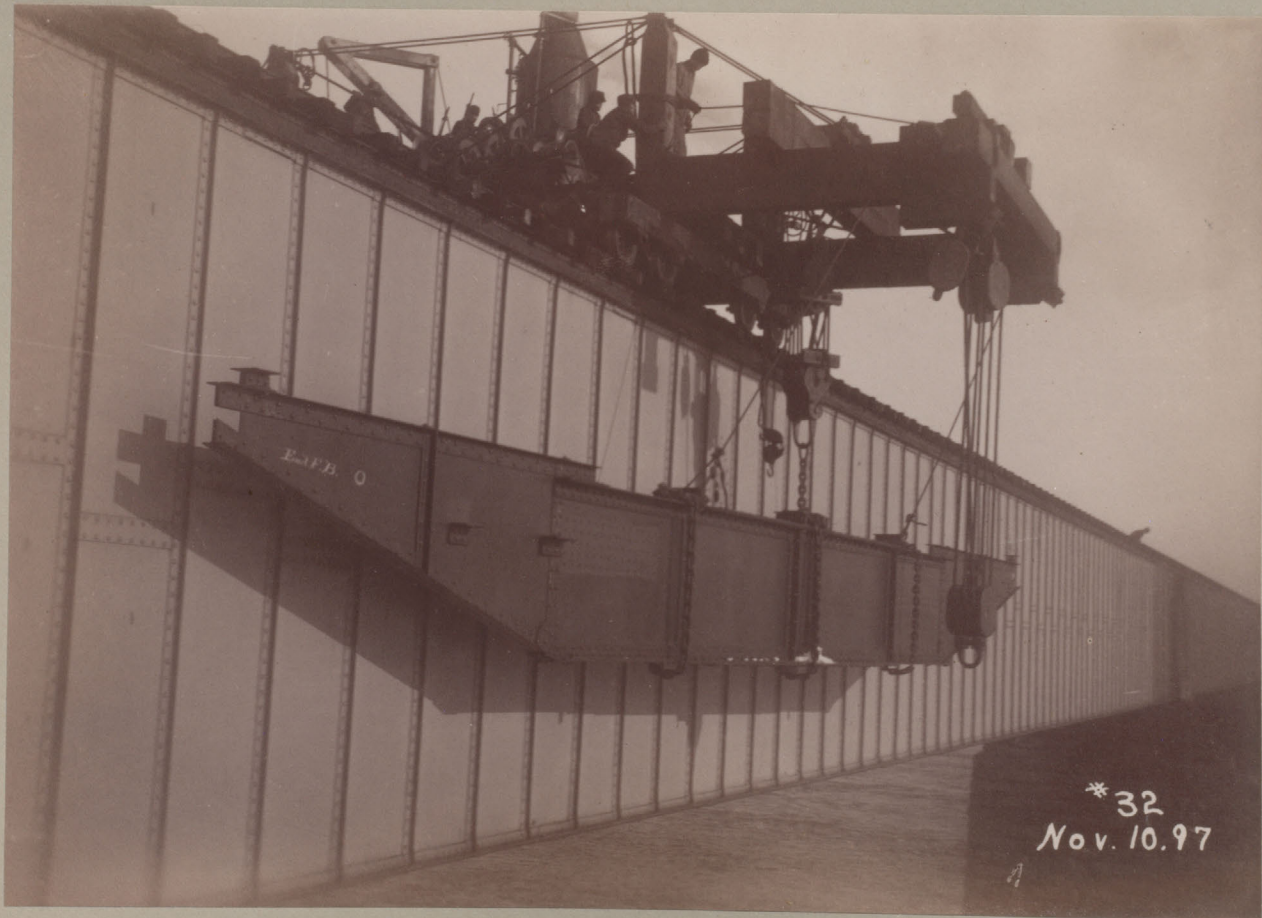
Traveller Carrying Out End Floor Beams Nov. 1897
