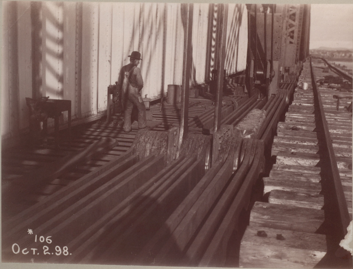
— Centre Joint - Bottom Chord - Centre Span —
