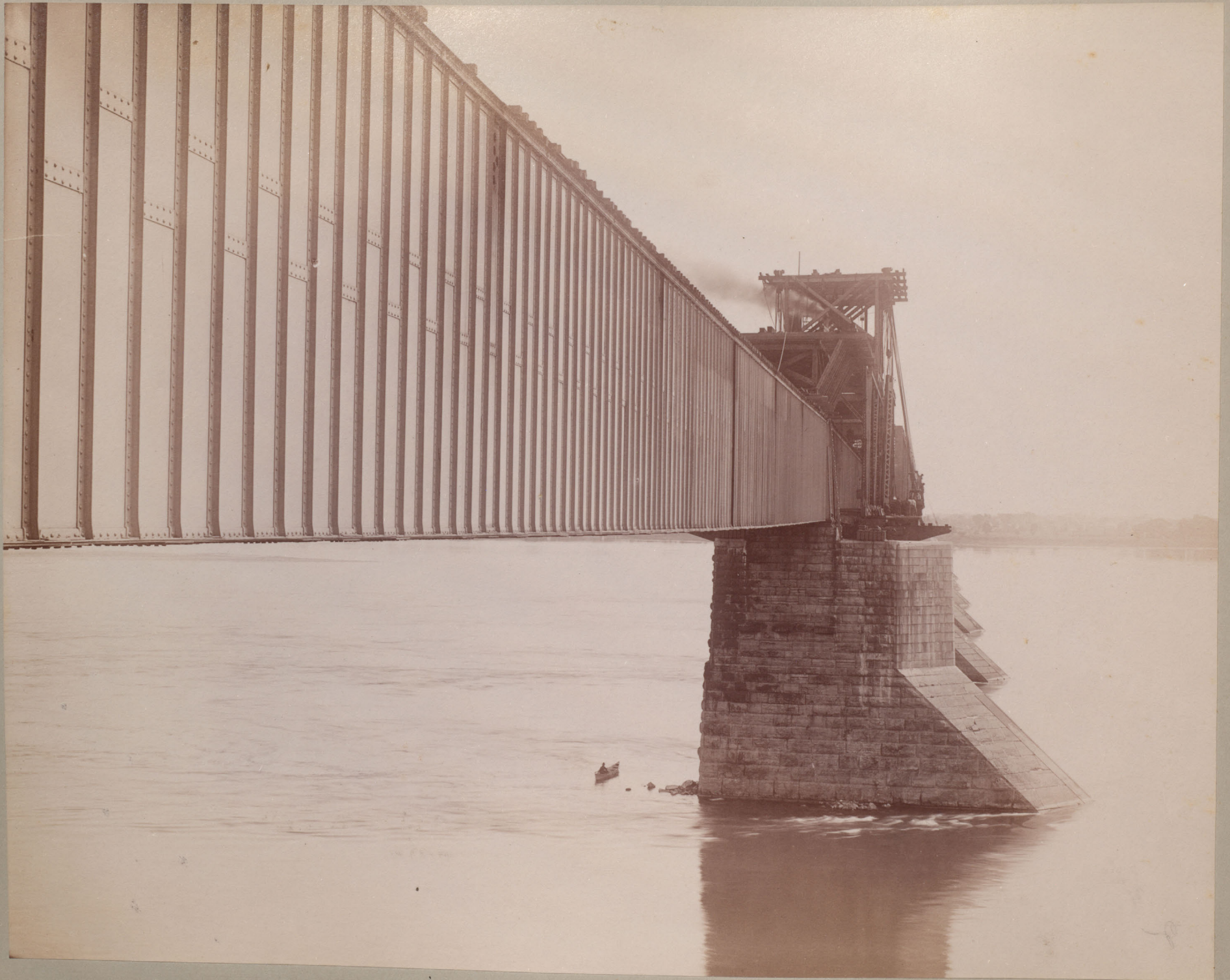
— pier N o 13. New Masonry Complete — — July. 1898 —
