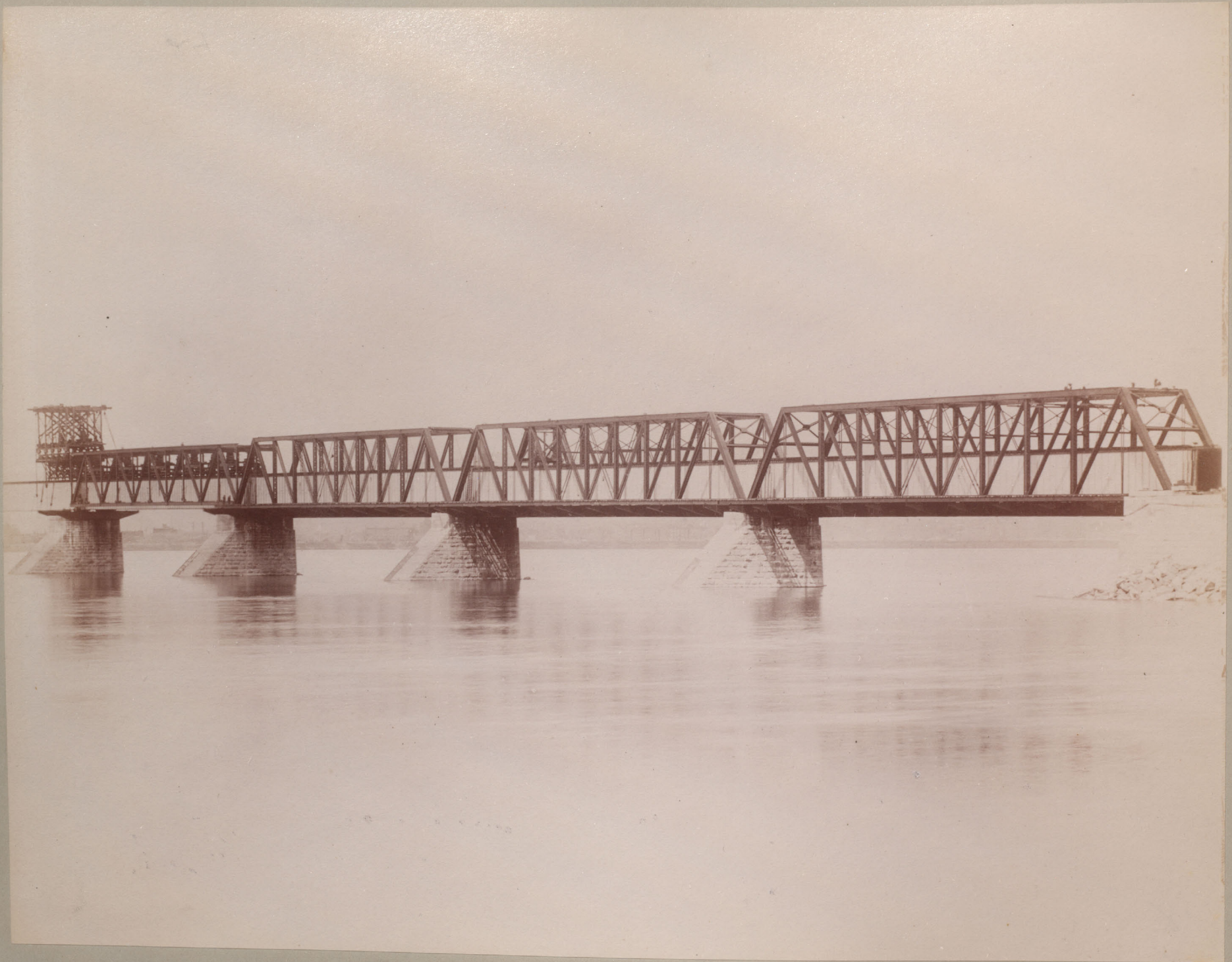
—Erection Truss in place Over Span 22—
